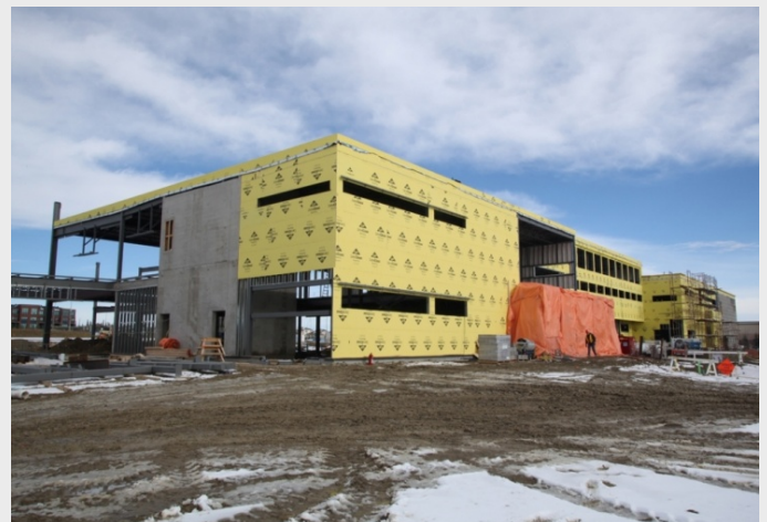
Looking northeast at the school's future main entrance.
