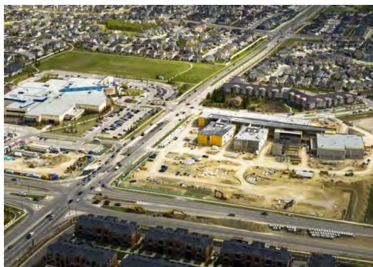
Looking south at the 69 Street Station site and West Calgary High School
