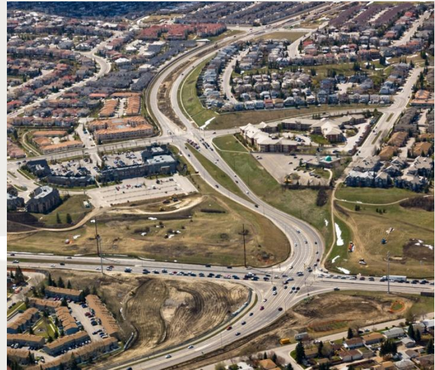
An aerial shot of the intersection at Sarcee Trail and 17 Avenue S.W.
