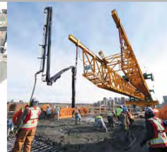
Workers pouring the Sunalta Station deck ▼
