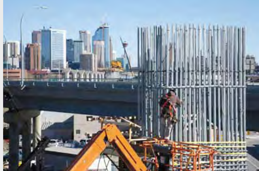
Worker constructing one of the 37 piers for the elevated LRT guideway
