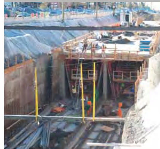
Workers constructing the LRT tunnel at 38 Street S.W. ▼
