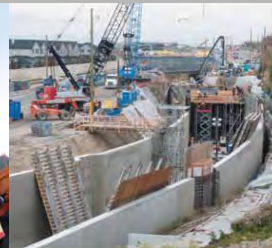
Constructing the tunnel under 17 Avenue S.W. to the 69 Street Station ▼
