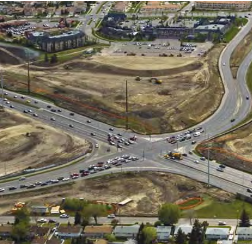
Sarcee Trail Interchange construction
